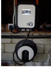
Sedan's L2 wall mount charger (left). Charging also controllable by cellphone (right):
